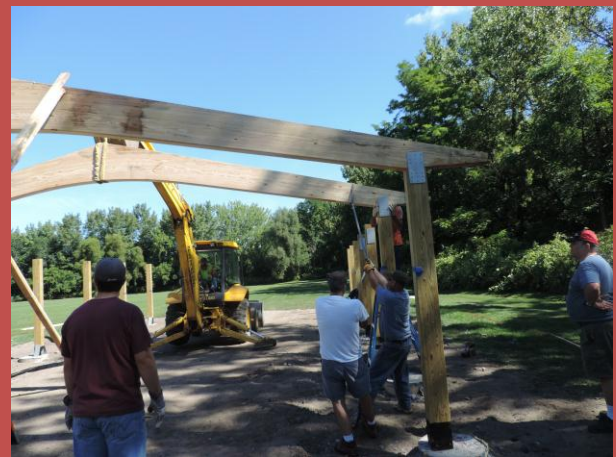
Second Truss is up!!
