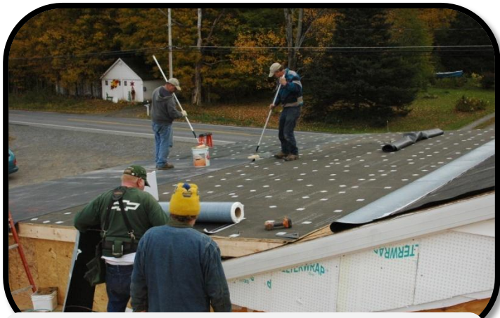
Lions Womer & Pike apply roof adhesive as Lions Putnam & Hodsoll work on another job (Oct. 10, 2009)
